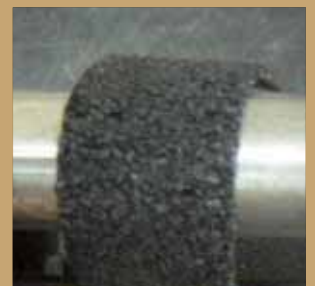
SBS – modified asphalt shingle with no cracking
